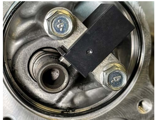
Grounding Brushes (typical)
